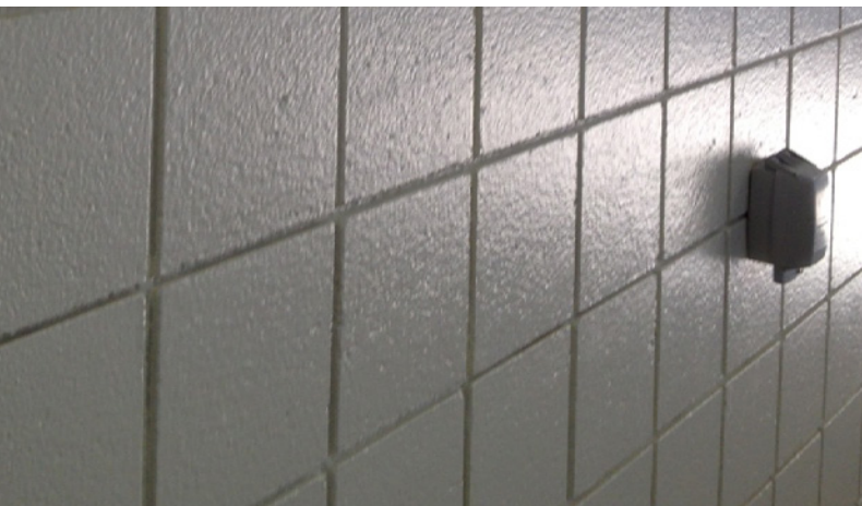
ABOVE : Spec-Finish Level II was used in stalls of the Animal Science Facilities.
