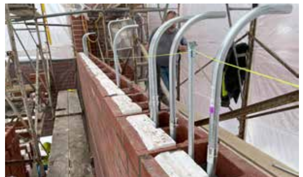
Utility routing in cores of HI-R-H units
