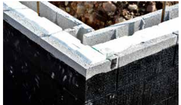
HI-R-H units were used to provide an insulated foundation
