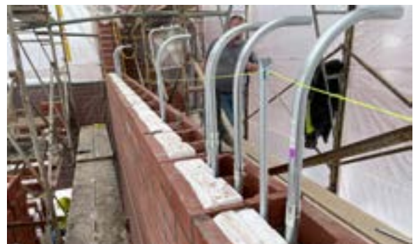
Utility routing in cores of HI-R-H units
