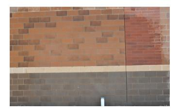
Cleaning walls during adverse weather conditions: Cleaning products will act differently in hot or cold conditions and drying times are influenced by wind conditions. Application of an acid based cleaner on a hot windy day requires reducing the area cleaned per section to allow proper removal of the cleaner. This can be a cause of staining if not addressed.
